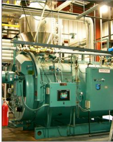
Figure 5.6 Gas-fired Super Boiler (Source: ITP 2008)
